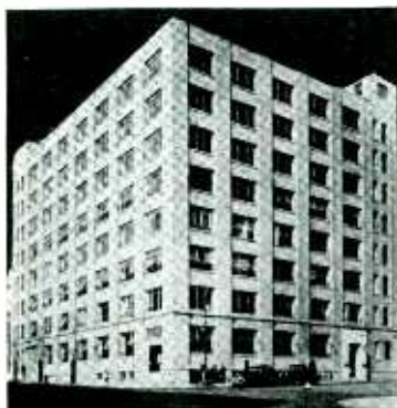
The New E.T.L. Building
