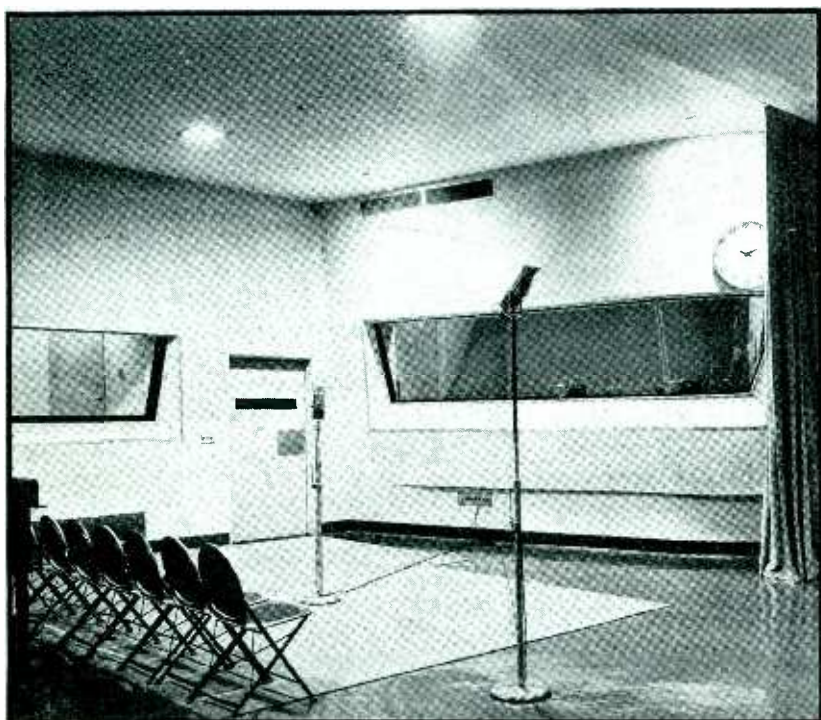
Left, typical small studio. The window of the control room is set at an angle so that annoying reflections to the engineer's eyes are avoided
