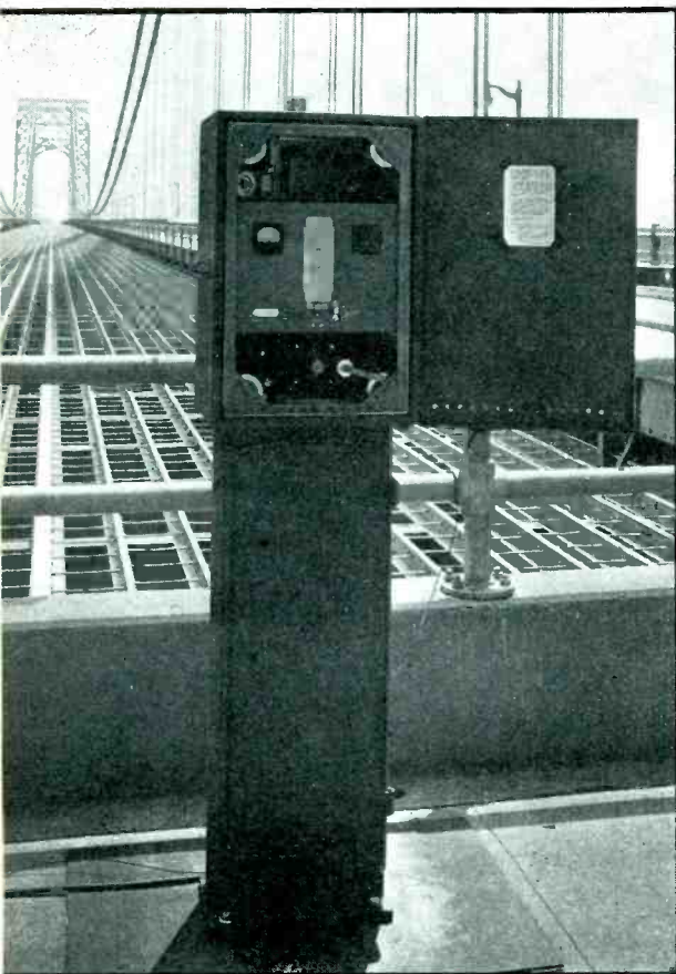
The transmitting equipment, shown above, includes a magnetic tape recorder and reproducer, which repeats a one-minute message
